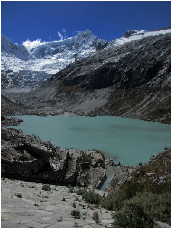
Figure 1. Laguna Llaca near Huaraz in 2013. Since the 1960s, the level of this lake at the foot of Nevado Ranrapalca (6162 m; background) was artificially lowered by about 30 m, greatly reducing the lake volume and the potential for large impact waves
