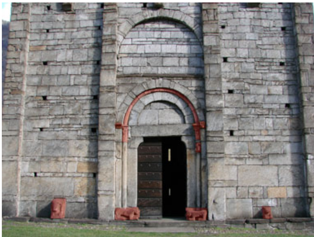
Figure 1. Lower part of western facade with main entrance of the San Nicolao church in Giornico. The soapstones are marked with red colour.
